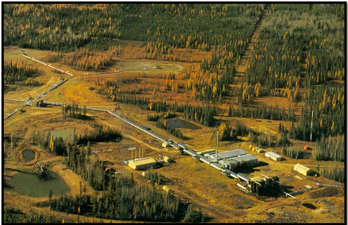
Figure 6.1. 3: Buffalo-Creek 10A Pilot facility (Norwest corporation report, 2008)
